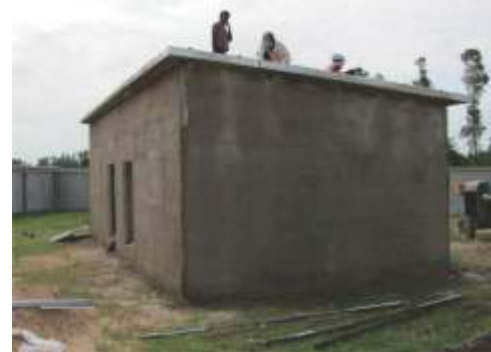
Above: Sunrise Orphanage's new office building taking shape
