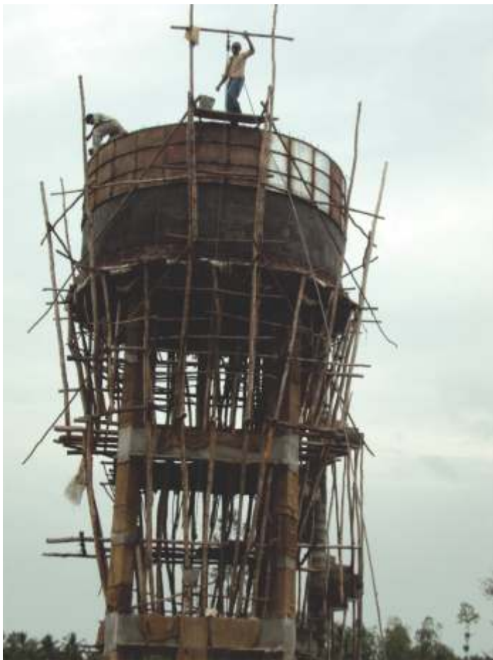
Water tower with tank going up
