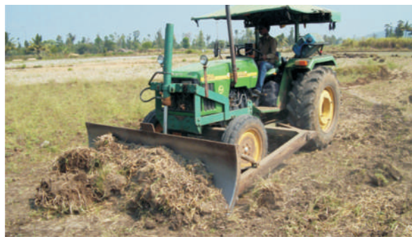
Bulldozers begin preparing the ground for construction
