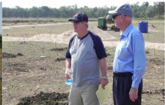
Doug Clark (left, in charge of Sunrise construction) and John Truscott (right, Asian Aid USA board chairman) check out the progress at the construction site
