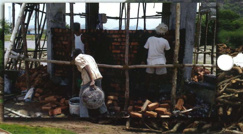
Below: Laying brick at water tower base
